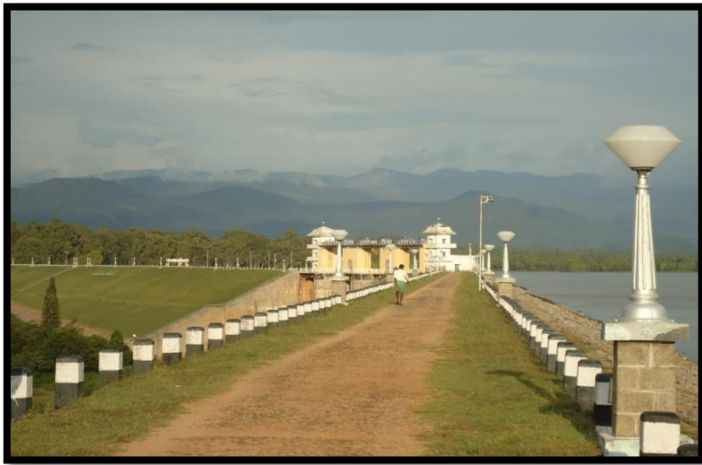
Pic: 5.1.1 (a) View of L/S & R/S Embankment of Suvarnavathi Dam
