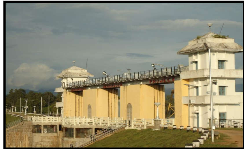
Pic: 5.1.1 (b) View of Center dam of Suvarnavathi Dam
