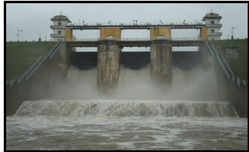
Pic: 5.1.1 (d) View of Spillway of Suvarnavathi Dam
