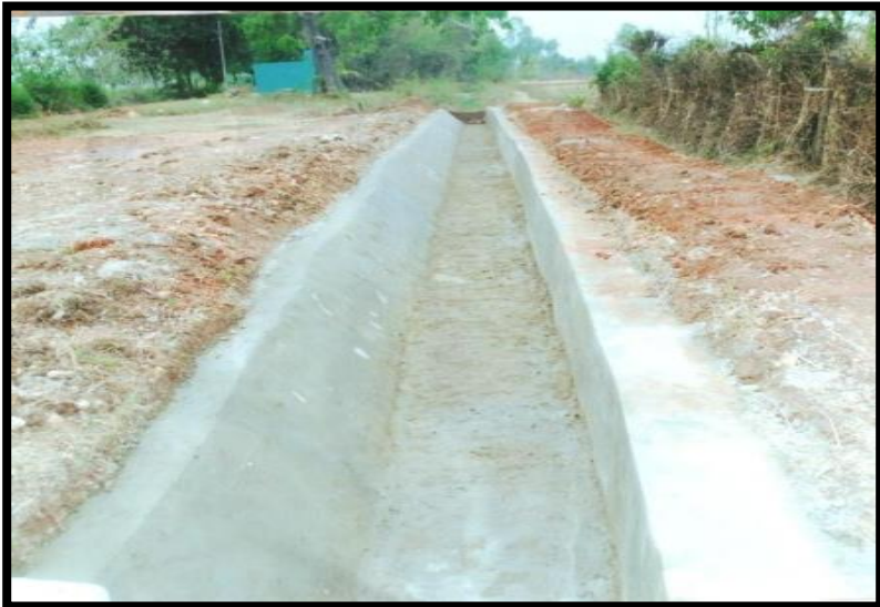
Pic 5.10. (c) Construction of Cement Concrete Field Channels
