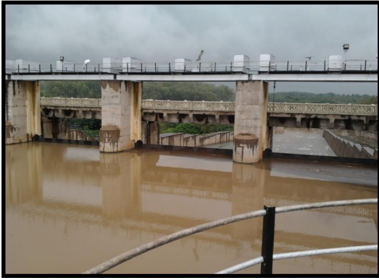
Pic: 5.1.2. (a) View of Chikkahole Dam
