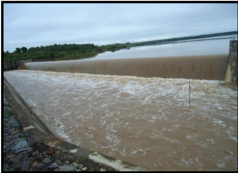
Pic: 5.1.2 (c) View of ungated spillway of Chikkahole Dam
