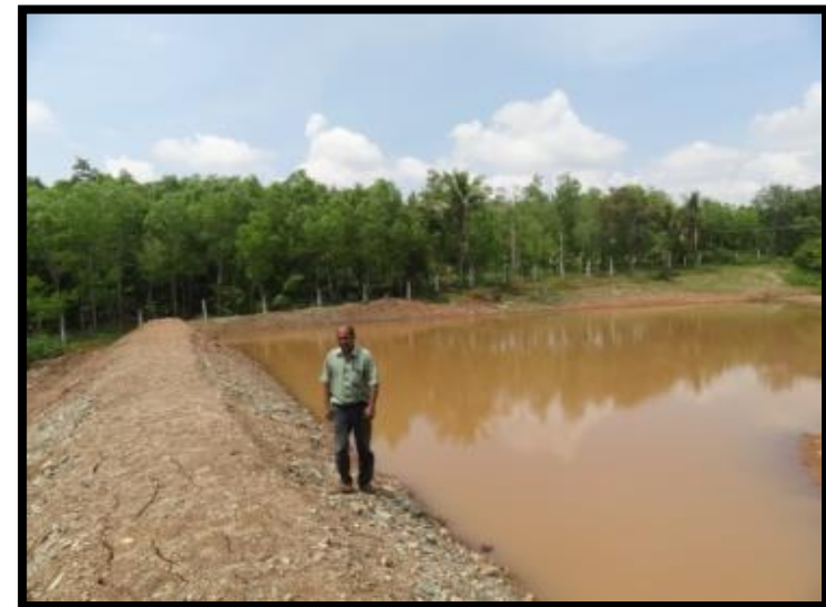
Pic: 5.6. (d) Construction of Nalabund across Nala at Downstream
