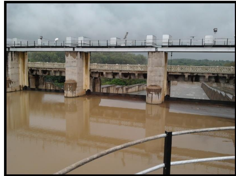
Pic: 5.1.2. (d) View of D/S of Chikkahole Dam
