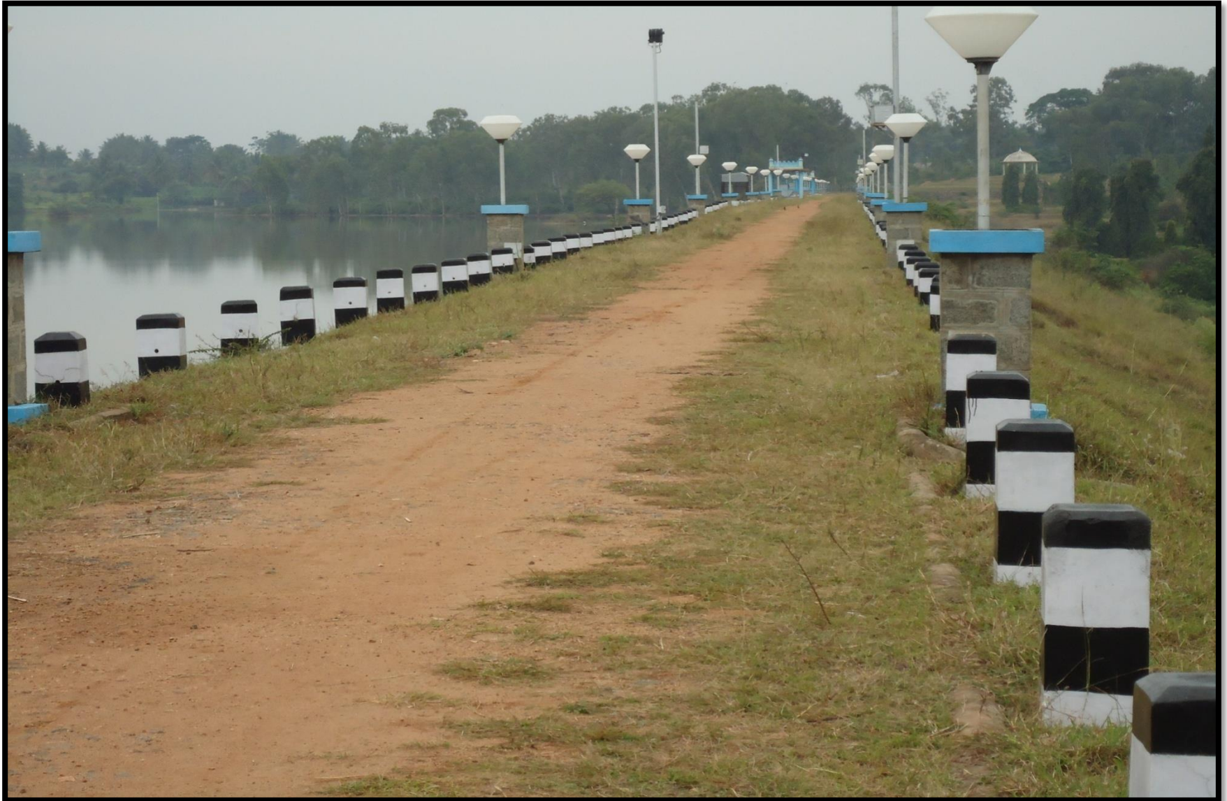
Pic: 5.1.2 (f) View of Top of Embankment of Chikkahole Dam
