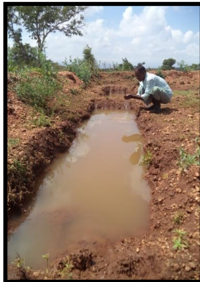
Pic: 5.6. (c) Insitu Rainwater Conservation through Trench cum Bunding
