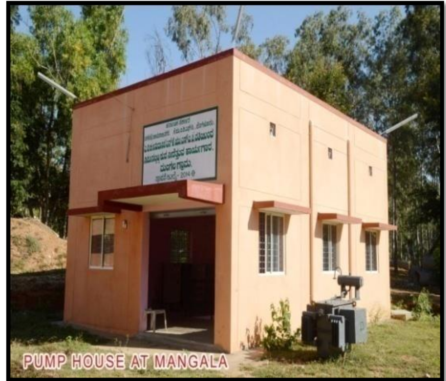
Pic 5.9.2 (b) Booster pump House at Mangala water Treatment Plant for Chamarajanagar Water Supply System
