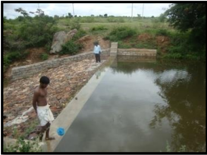
Pic: 5.6. (a) Construction of Check Dam across drainage lines
