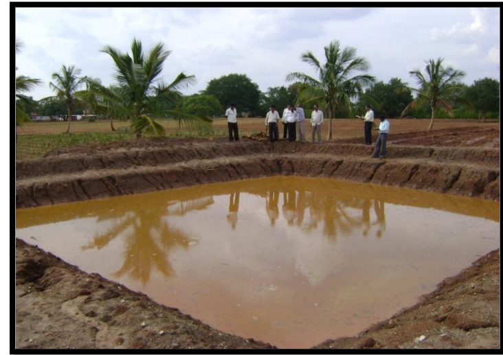
Pic: 5.6. (b) Construction of Farm Pond for Harvesting Rainwater
